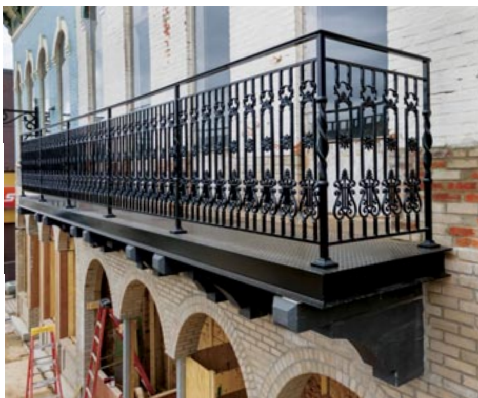
The ornate balcony is supported by newly-installed wooden brackets and masonry.
