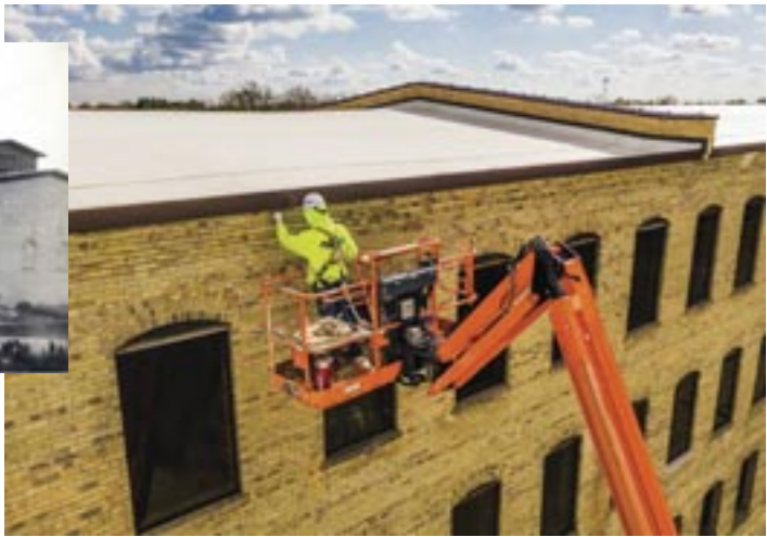
An astonishing 3.2 million vintage bricks were repaired or replaced and tuckpointed as part of the extensive restoration of The Mill's 120-year-old exterior.
