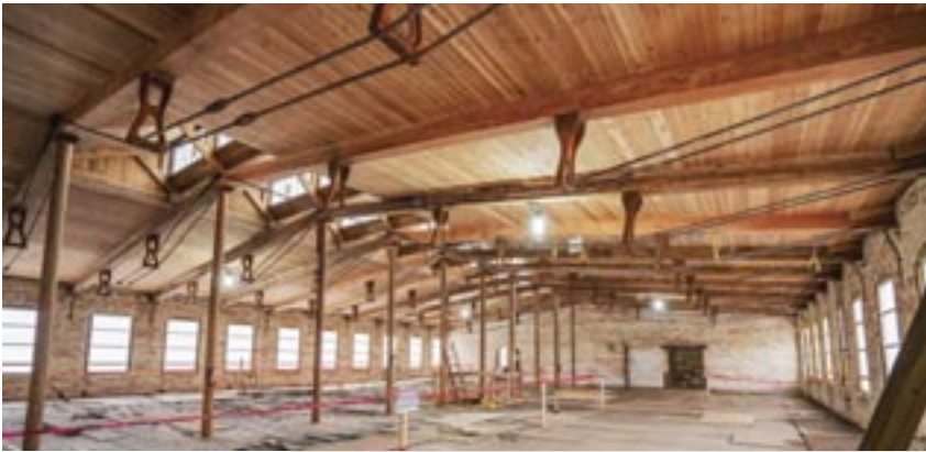
A section of the Mill's interior shows the extensive prep work required before reconstruction. This includes stripping the wood and other surfaces of 8 layers of lead paint. Plans call for the replacement of 1500 windows with new ones that are historically correct.
