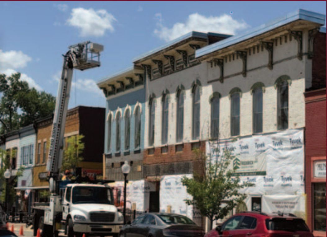
The crane was needed for work on the second story as well as a full restoration of the ornamental cornice that supports the roof overhang.
