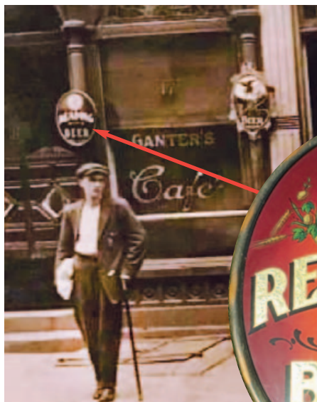
Corner sign of reverse-painted glass with gold leaf lettering, 16.25 x 20.25 in., by The John L. Dawes Mfg. Co., Pittsburgh, PA, c. 1900. Collection of Chris Watt. The sign is seen hanging here from a cast iron support post at Ganter’s Café on Sixth Street in Reading, which operated until just before Prohibition. The building has long since been demolished. Courtesy of Mike Pentz.
