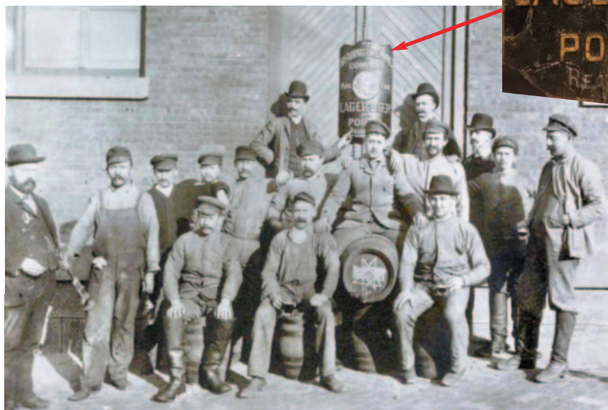
Original photo of Reading Brewing Co. workers posed outside of the brewery, c. 1890s.
