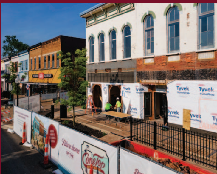
The extensive façade restoration began in March and considerable progress had been made at the time of this photo on May 16. This endeavor first required extensive and historically accurate architectural plans (right).
