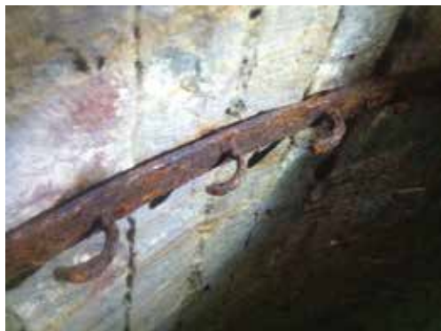
Closeup of the Nunning cellar's iron support bands (shown at left) with hooks, reportedly used to hang harvested hop vines.
