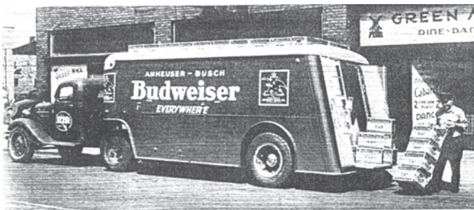
Above: This specially built semi-trailer is used in city delivery of Budweiser by the Sam J. Izzo Co., Saginaw, MI. The roof well is for empty cases. The trailer replaces two conventional trucks.
