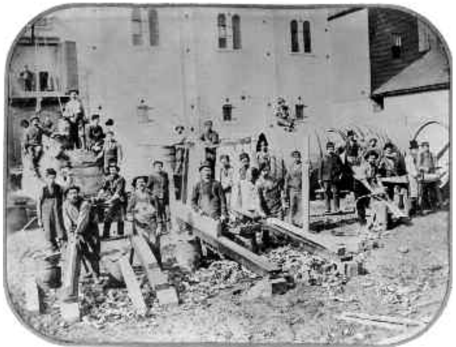
Twenty-six coopers were working outdoors in 1878. They are hand-building huge 10 barrel stock tanks. The "normal" product, wooden half- and quarter barrels are being used as lifts for the froe users in the left foreground.
