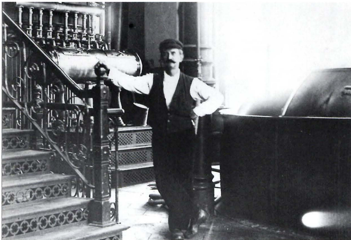
A self-assured head brewer posed before the eight-tap grant, where wort was collected from different points below the lauter tun. The combined wort then ran into one of two brewkettles.
