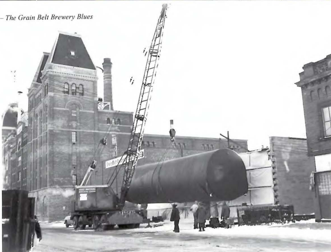
Major construction was started in the summer of 1962. One of nine 1,265 barrel glass-lined tanks were being installed in January 1963 (top). Ground was broken in February 1963 for a $250,000 addition to the keg house for storage of keg beer (bottom). Photos in this article are by Mike Hajicek.
