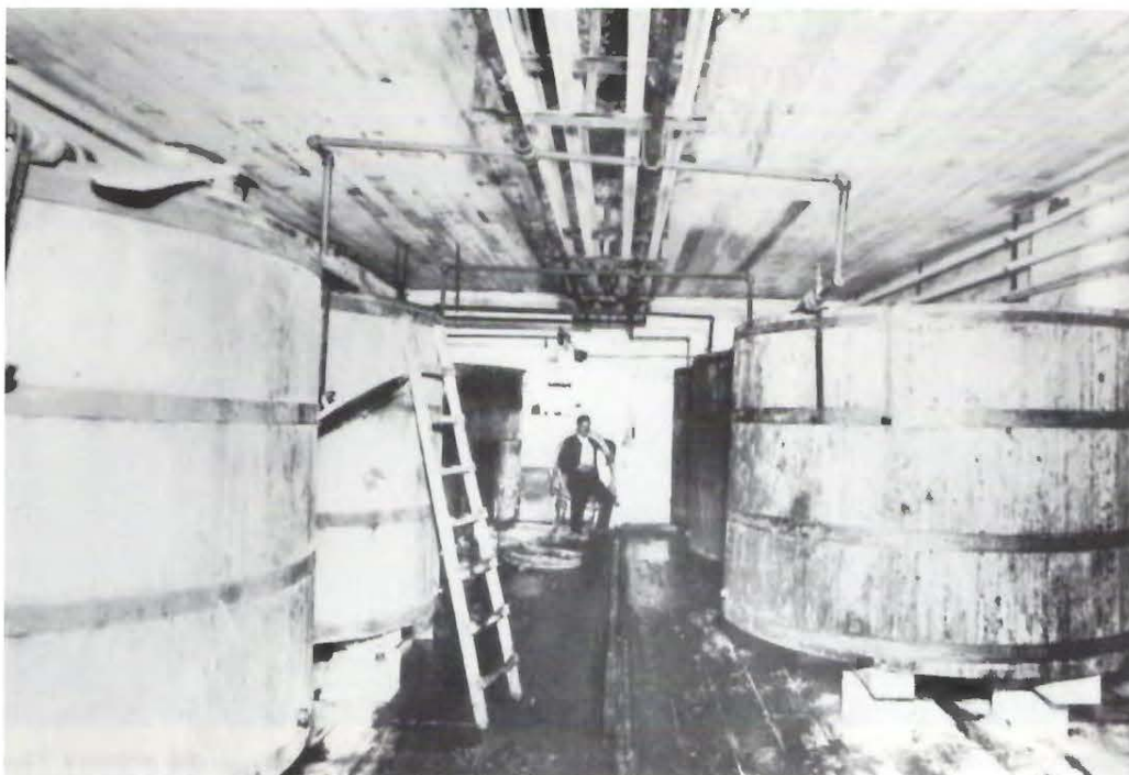
Above: Open fermenters are of customary flat-bottom design and have a capacity of about 80 barrels. Cellar man in background is holding several coils of two inch beer hose. Pipes on ceiling and at side are for circulating ammonia refrigerant. Below: Well-maintained engine room has a steam-driven ammonia compressor to cool storage cellars.
