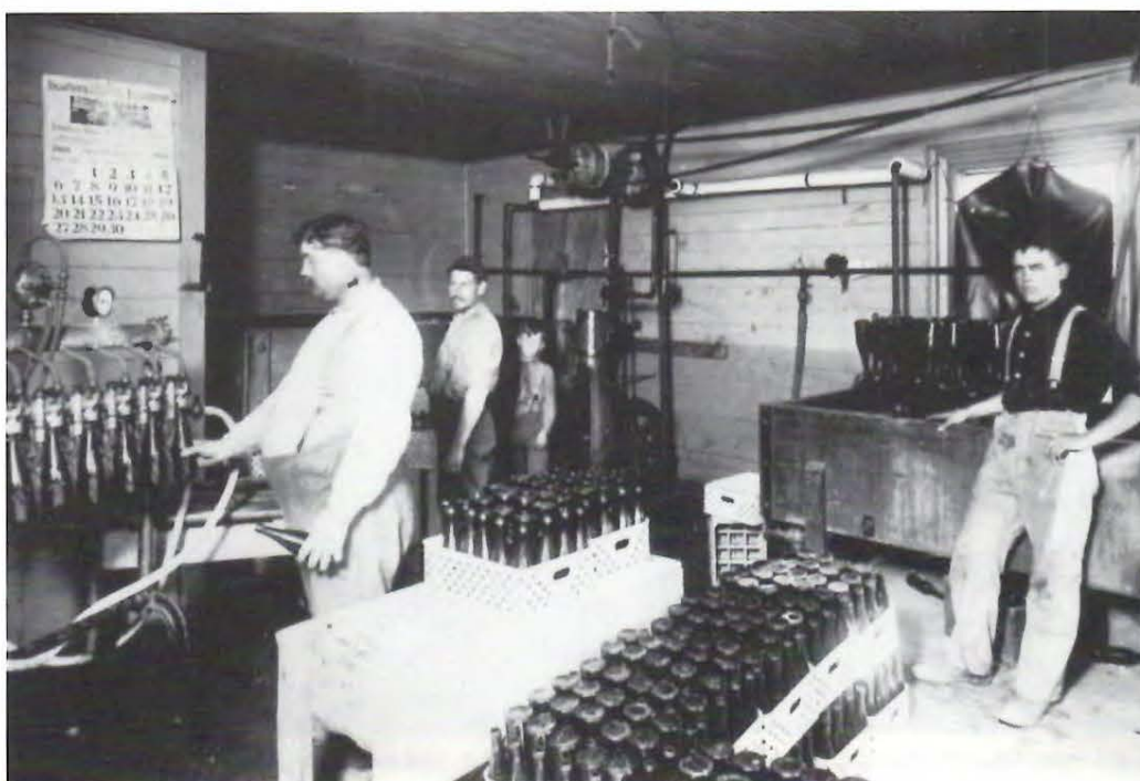
Above: Racking cellar is cramped but contains good cooperage. Coils on ceiling show frost condensation on pipes containing circulating expanding ammonia. Below: Bottle shop is equipped with straight-line filler and simple basket pasteurizing tank. Boy in background standing in front of beer pump seems smaller than those usually seen in brewery group photos. Wall calendar shows September 1908. Original photos belong to Norman Yogerst.
