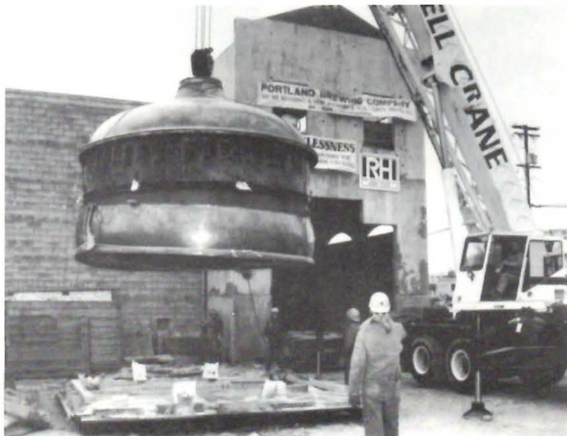
Above: Brewkettle from Germany being moved into new Portland brewery.
