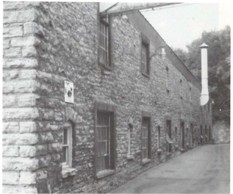
Top left and above: Original brewery limestone construction can still be seen on the southwest corner of the brewhouse. Many of the window openings have the original stone arches and sills. Wooded area in background is Dayton's bluff, source of stones. Bottom left and below: Road leads down to bottom of gully where railroad spur still runs. Buildings on other side of Minnehaha overpass are powerhouse and a warehouse. Culvert was known as Phalen creek long ago.
