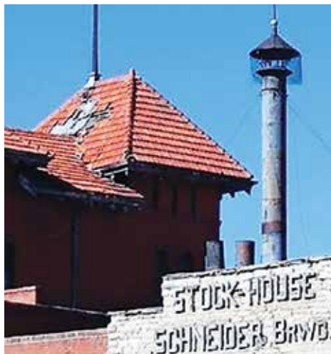
Close up of the stock house, with the brewery tower in the background and roof tiles in obvious need of repair.
