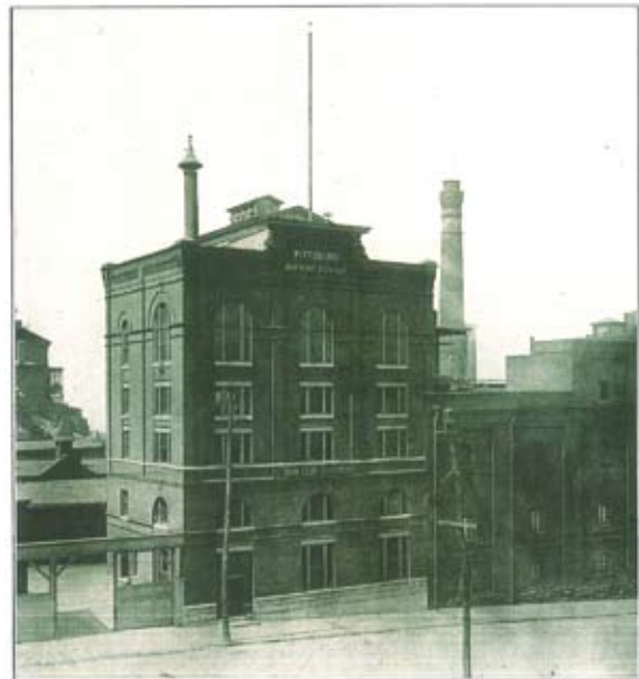
WINTER BRANCH, PITTSBURGH BREWING CO., PITTSBURGH, PA. OTTO C. WOLFE, ARCHITECT W.M. MILLER & SONS CO., BUILDERS
